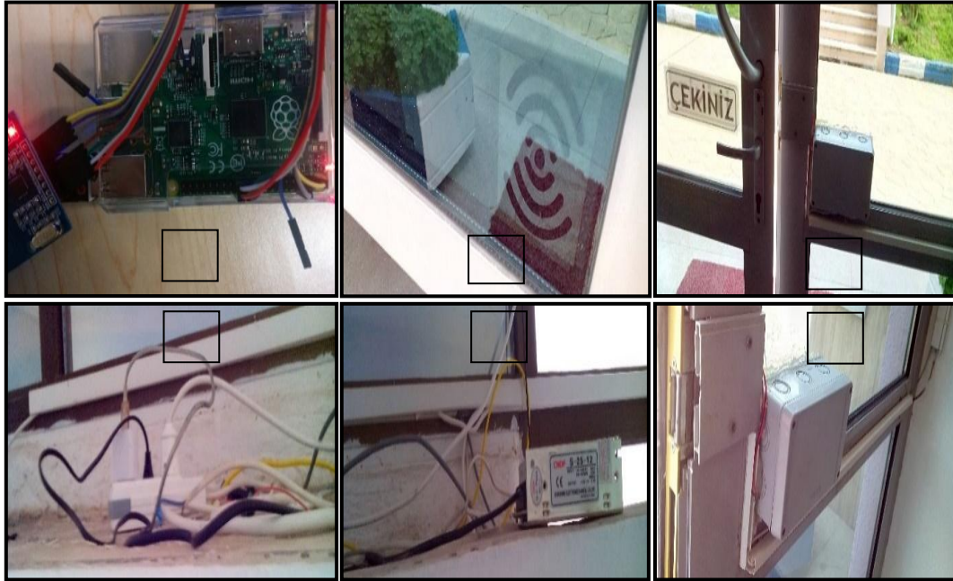
Figure 16. Actual implemented system of this research work (a single section only). Section A shows the connection of a single SN unit with a Raspberry Pi and an MFRC522 sensor. Section B, C and F shows one of these units mounted in a door. Section D and E shows the power and internet connection to this unit.
