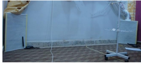
Fig.7 Photograph for supply diffuser type-III illustrated the location at test room
