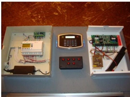
Fig.15 Termination in the units
