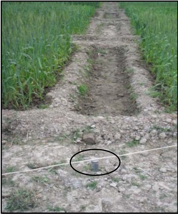
Fig 5: Installation of piezometers (2008/09) at 30 locations to monitor changes in groundwater during the season.
