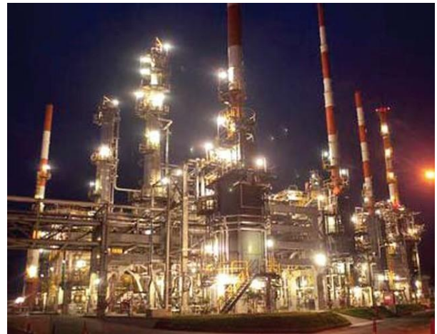
Fig 6.4: Power plant lights
