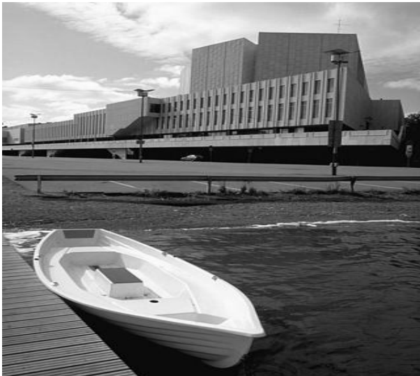
Fig 2: The image of a canoe and a building
