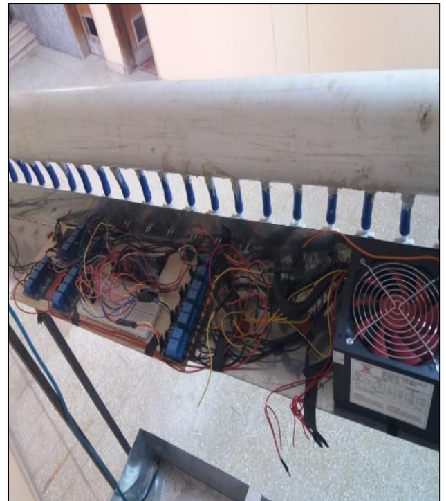
Fig.6.the internal design of the iron structure of fountain.
