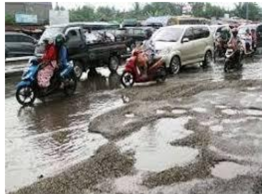
Figure 2.1. Congestion is caused by road damage. Source: (tribunjabar.com)
